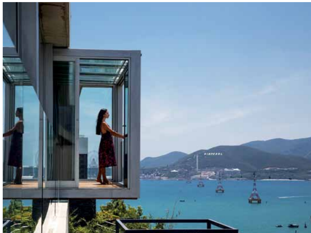
The cantilever extension adjoining the bedroom.
